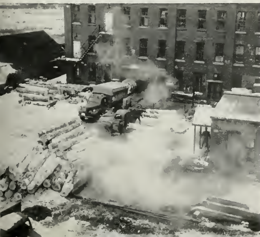
Winter weather fails to interfere with operations at RCA Victor cabinet factory in Owen Sound, Ontario.
